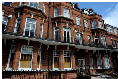
Elm Park Gardens Basement conversion into Key Worker units
